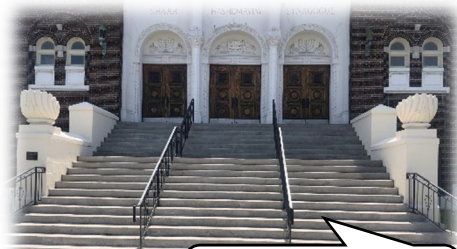
Shaar Staircase after Power-Washing
