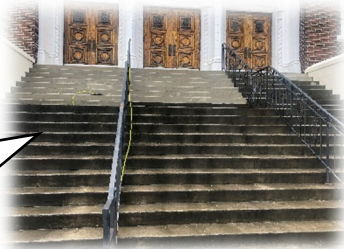
Shaar Staircase during Power-Washing
